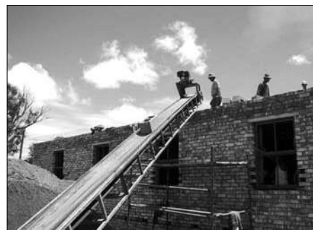
Simple 'made-in-house' conveyor belts to carry goods to a higher level.
